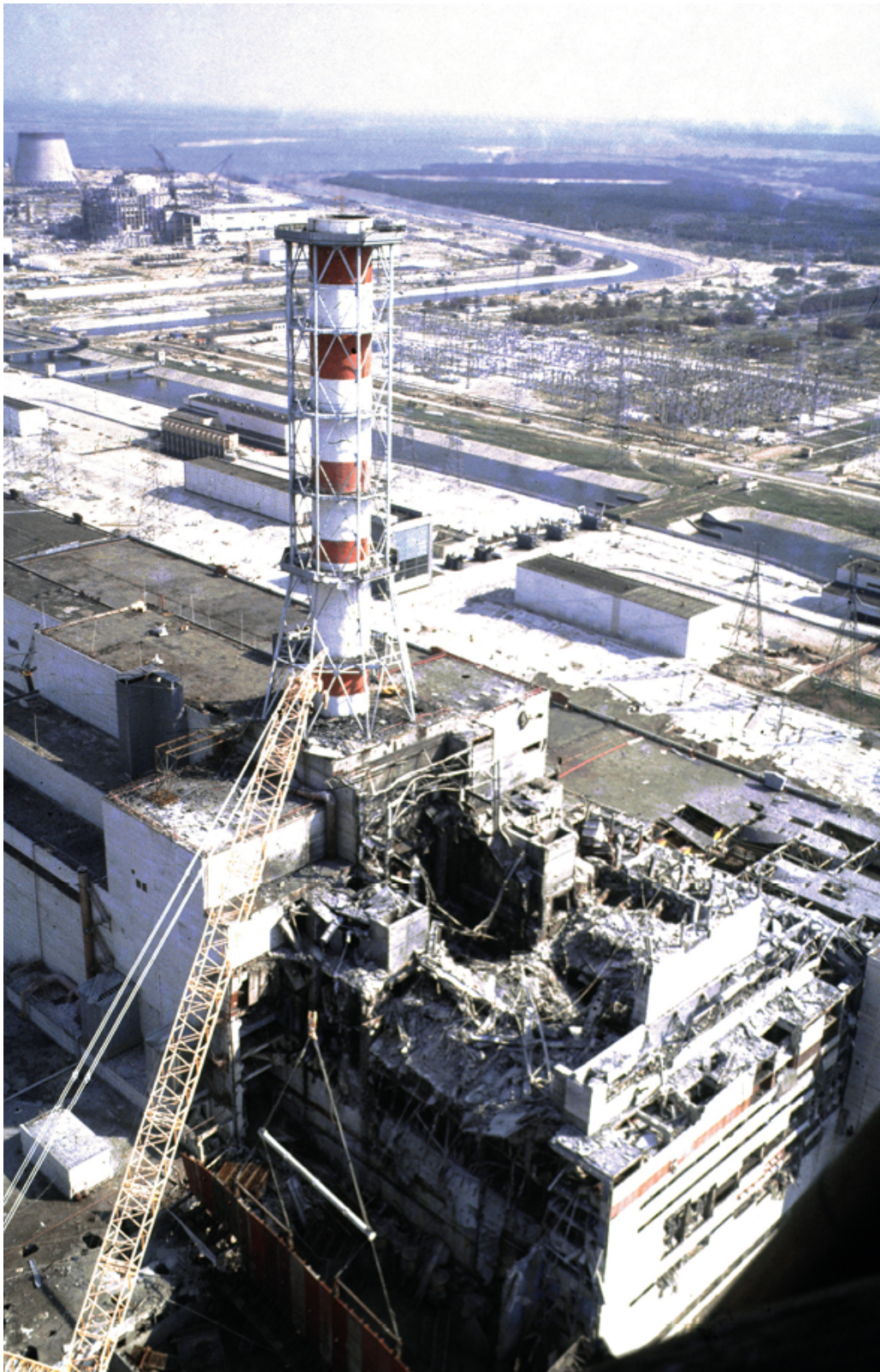
Figure 7.4: The Chernobyl nuclear power plant three days after the explosion in April 1986.
